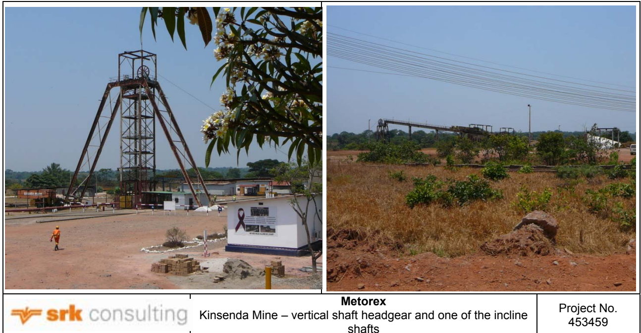
Figure 5.2: Kinsenda Mine – vertical shaft headgear and one of incline shafts
