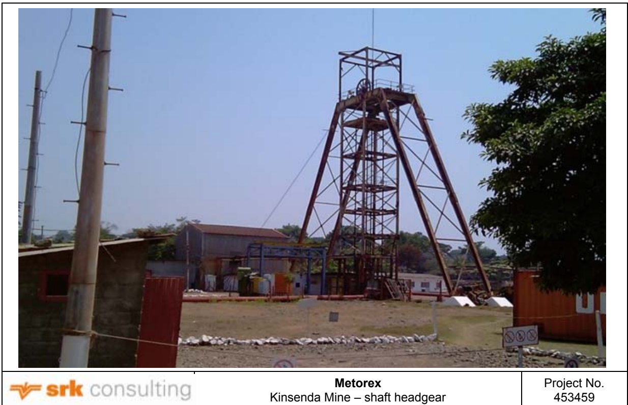
Figure 5.22: Kinsenda Mine – shaft headgear
